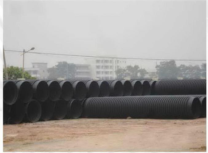
The transport of Technoplast pipes is very easy as they are easily moved due to the low weight. Normally the pipes can be unloaded and transported to the trench by an excavator, which is anyway present on site. For the storage of the pipes and fittings it is absolutely necessary that they are stored on an even ground, free of stones and sharp-edged objects, so that point-load is avoided.
